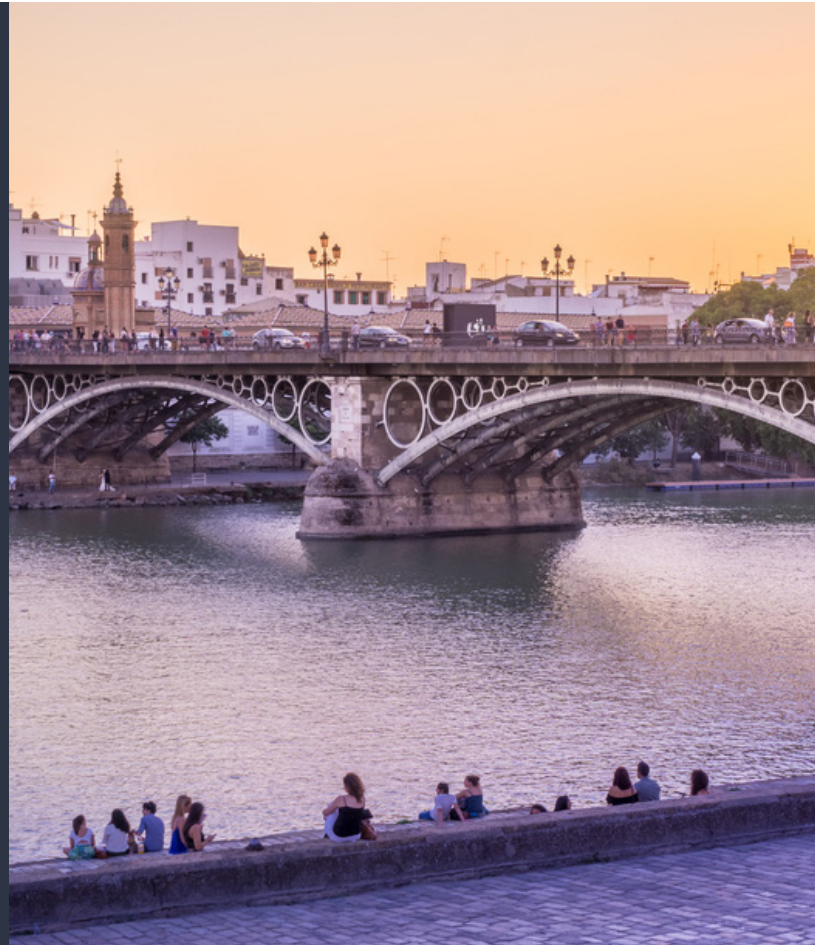
▲ ISABEL II BRIDGE
